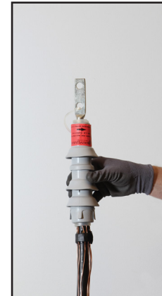
3. Support Core Removal
