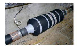
A Click Fit joint type CFJ(X) with designation "-OF" provides a possibility to splice and store the integrated optical fibers from the extruded (extra) high voltage cables within the metal casing. Suitable for Multimode and Single Mode optical fibres.
