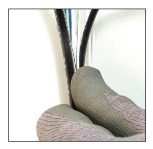
Cut the strength yarns to desired length as specified by local practices or the closure manufacturer.
