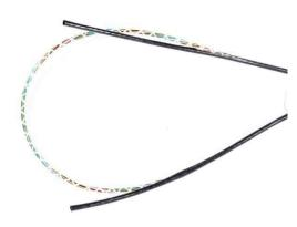
**6.18** Use your snips or other approved tool to remove the yarns, water blocking material and rip cords.
