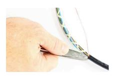
**6.15** Pull the rip cords down the jacket until you reach the desired length of sheath to be removed.
